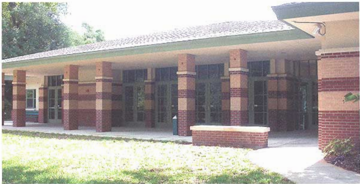
Recreation Center south elevation fm the tennis courts
