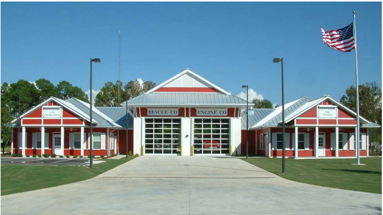
Callaway's Public Safety Building construction completed in 2009
