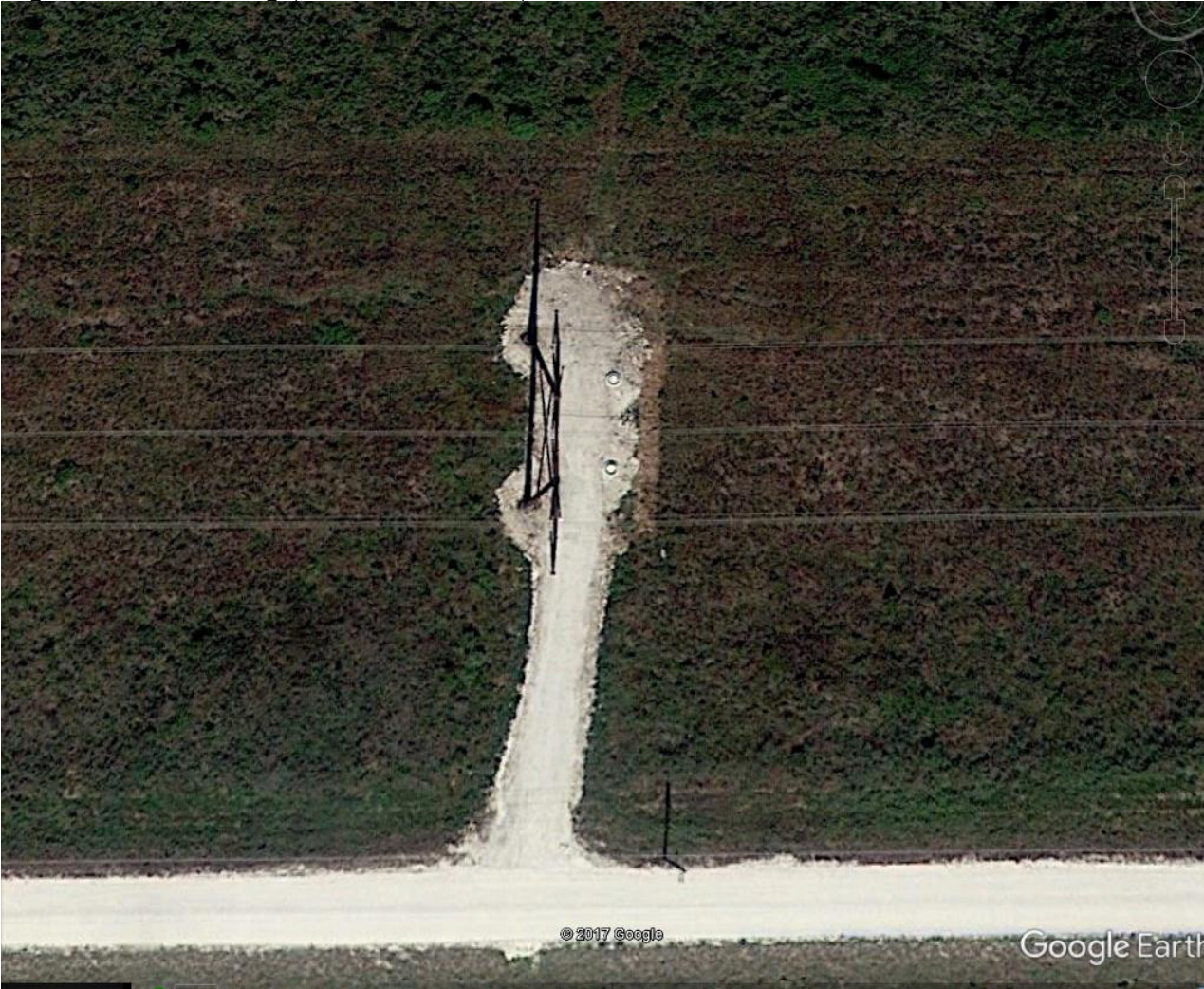
Figure 9. Aerial Image, L-5 North Levee, Power Pad
