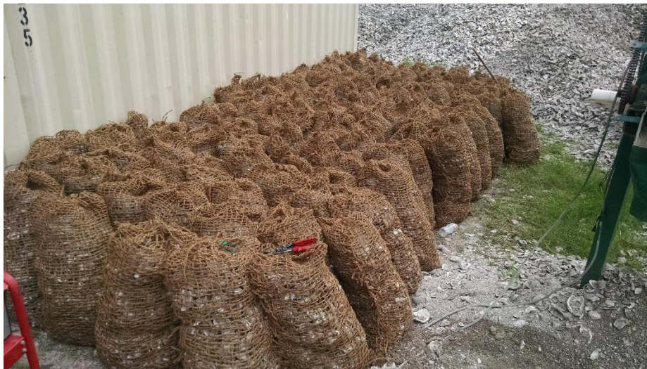
Figure 1: Biodegradable coir fiber bags, filled with oyster shell material, waiting to be moved to the barge that will take them out to the restoration site.
