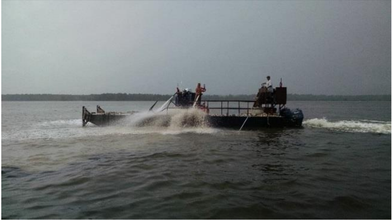
Figure 7: High powered water hoses were used to wash and blast the shell off the barge onto the reefs.
