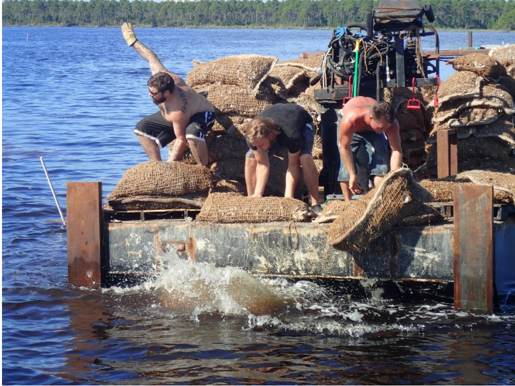
Figure 3: Biodegradable coir fiber mesh bags being pushed off the barge to be placed on the edge of the oyster reefs.
