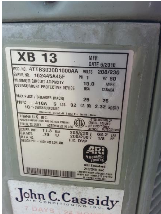
AHU-1 (2.5 tons) - 2010
