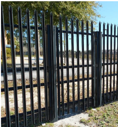
Photo of existing perimeter AT/FP high security fence surrounding bldg. 1822
