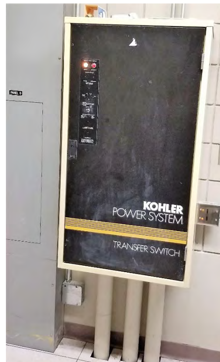
AUTOMATIC TRANSFER SWITCH (ATS)
