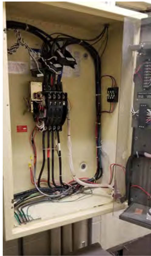
AUTOMATIC TRANSFER SWITCH (ATS)
