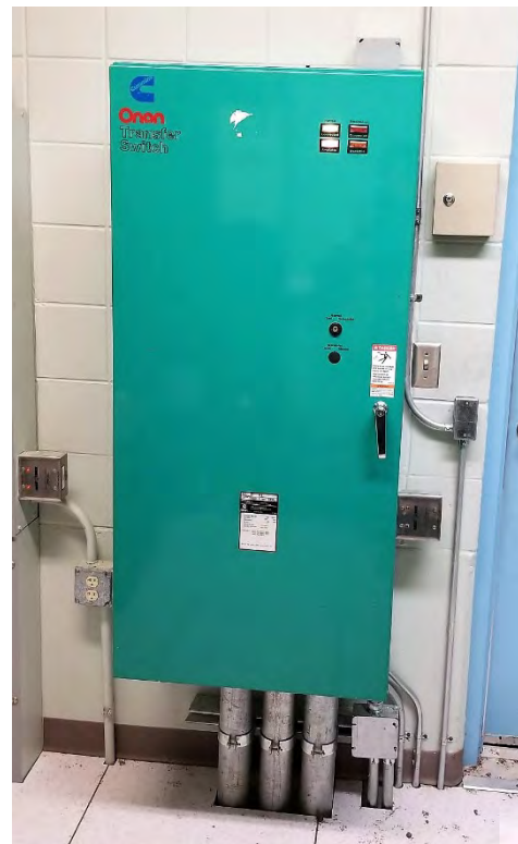
AUTOMATIC TRANSFER SWITCH (ATS)
