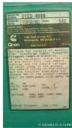
AUTOMATIC TRANSFER SWITCH (ATS)
