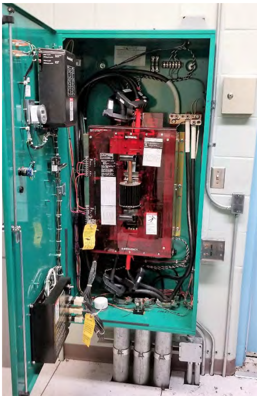
AUTOMATIC TRANSFER SWITCH (ATS)
