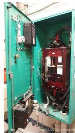
AUTOMATIC TRANSFER SWITCH (ATS)
