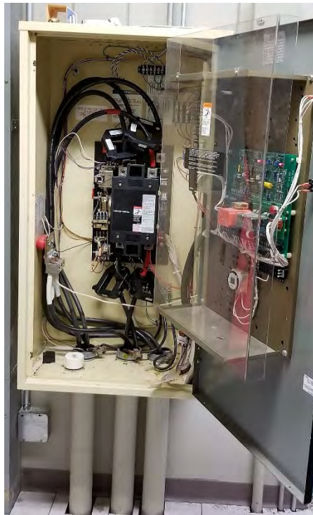
AUTOMATIC TRANSFER SWITCH (ATS)
