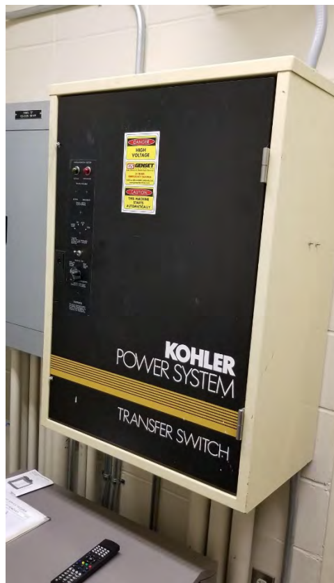
AUTOMATIC TRANSFER SWITCH (ATS)
