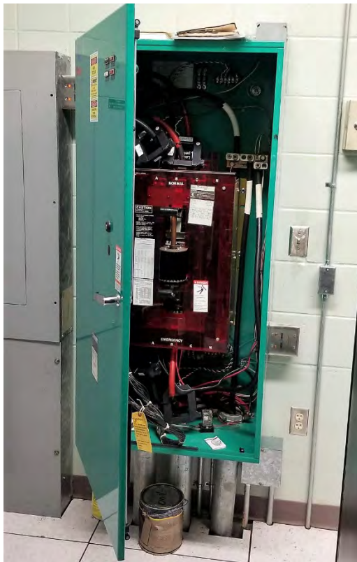
AUTOMATIC TRANSFER SWITCH (ATS)
