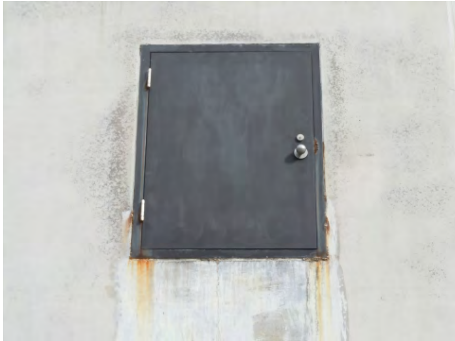
Photo #13 - South Elevation, West End
