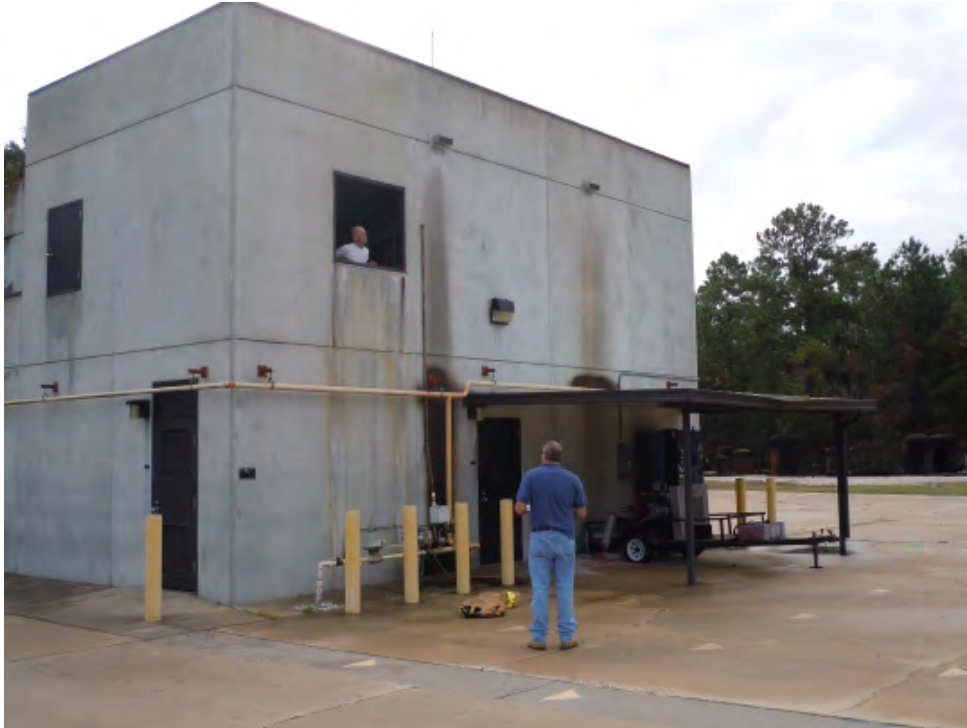
Photo #3 - West Elevation
