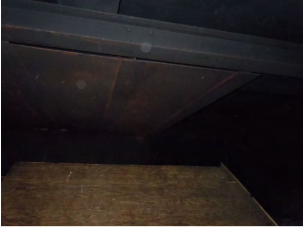
Photo #19 - Scenario Room #1 (NW) Ceiling Plates
