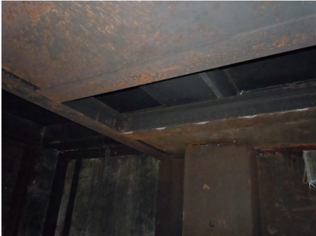
Photo #25 - Scenario Room #3 (SE) Ceiling Plate Removed
