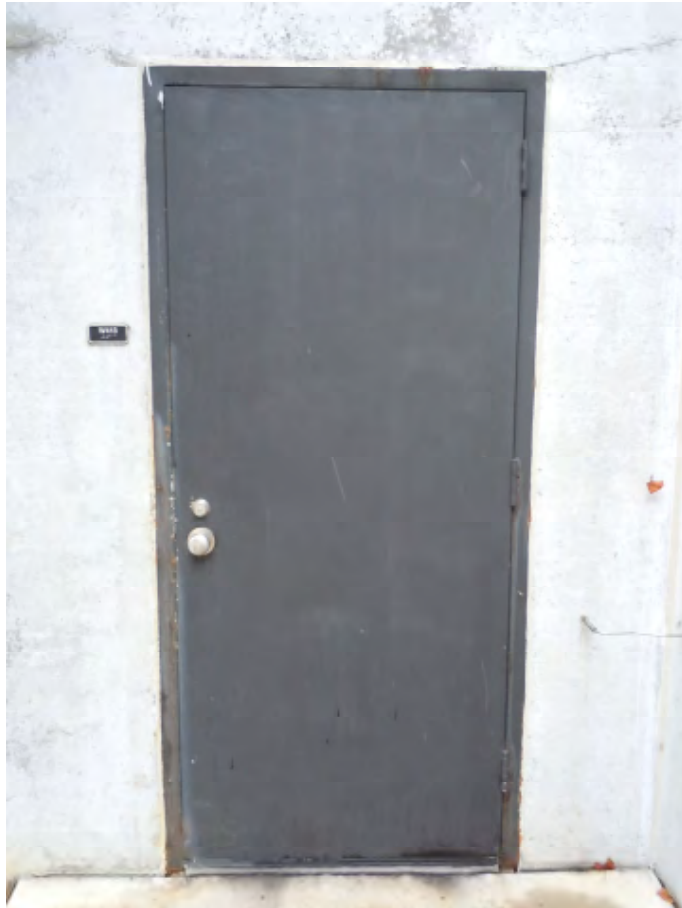
Photo #5 Exterior Door, East Elevation
