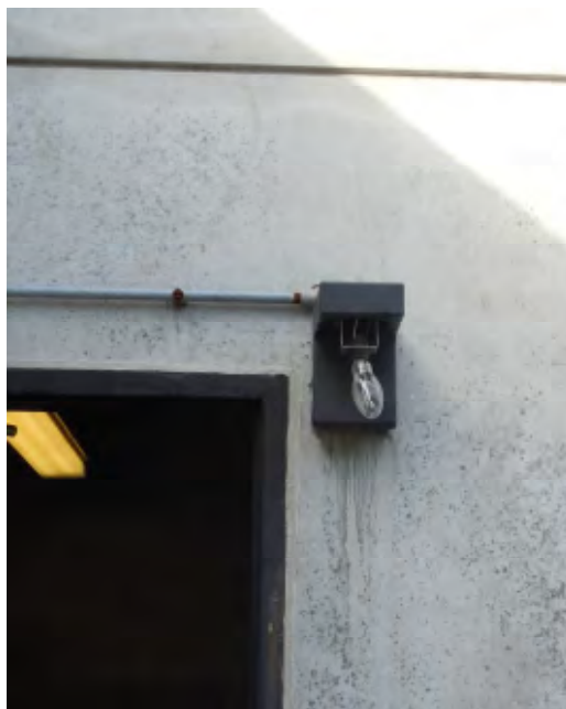
Photo #16 - Low Roof, North Side, Looking West
