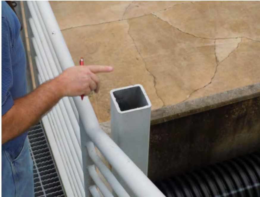
Photo #11 - Exterior Stair
