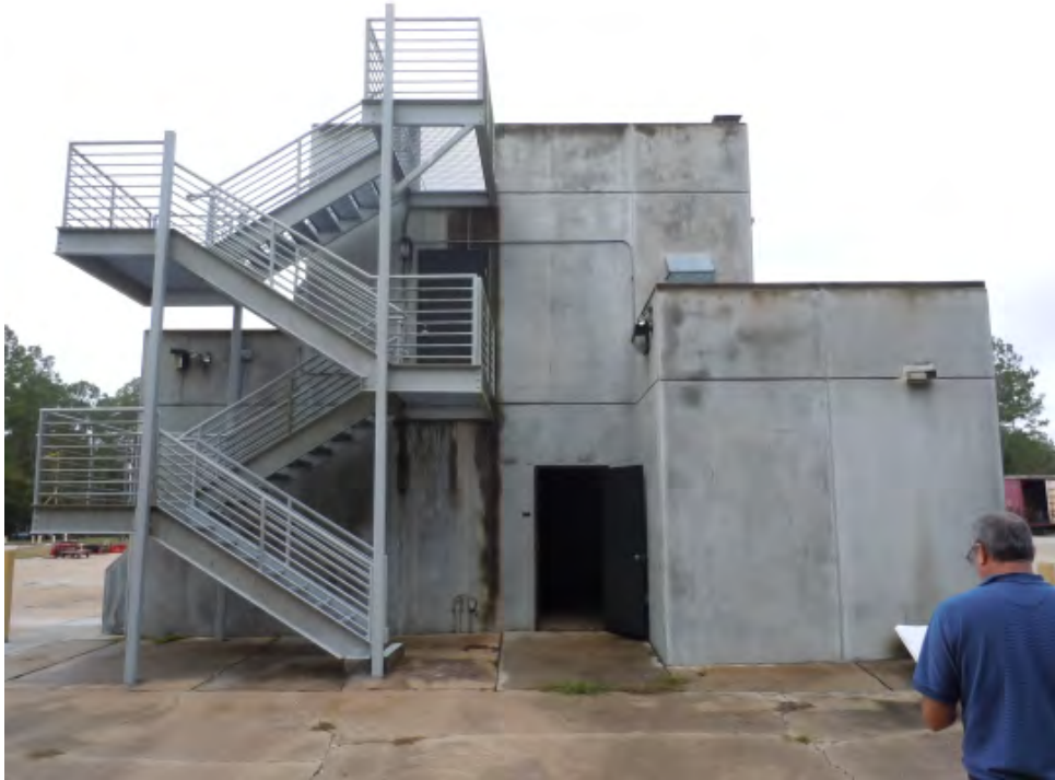
Photo #1 - East Elevation
