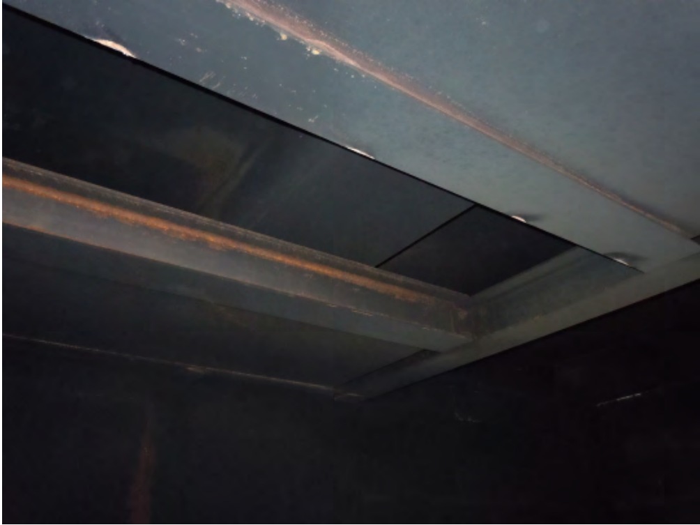
Photo #27 - Scenario Room #4 (SW) Ceiling Plate Removed
