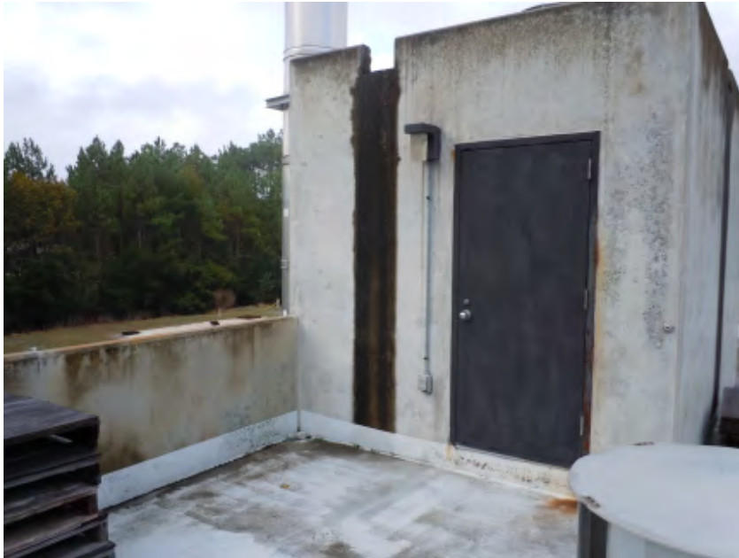
Photo #7 - High Roof, South Side
