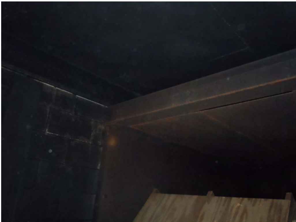
Photo #20 - Scenario Room #1 (NW) Ceiling Plates
