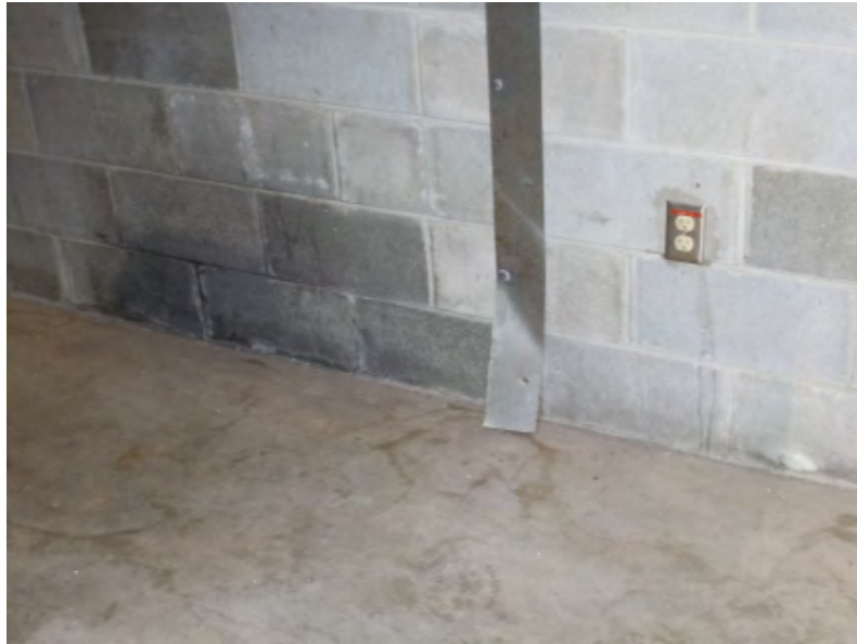
Photo #17, Second Floor Corridor, North End
