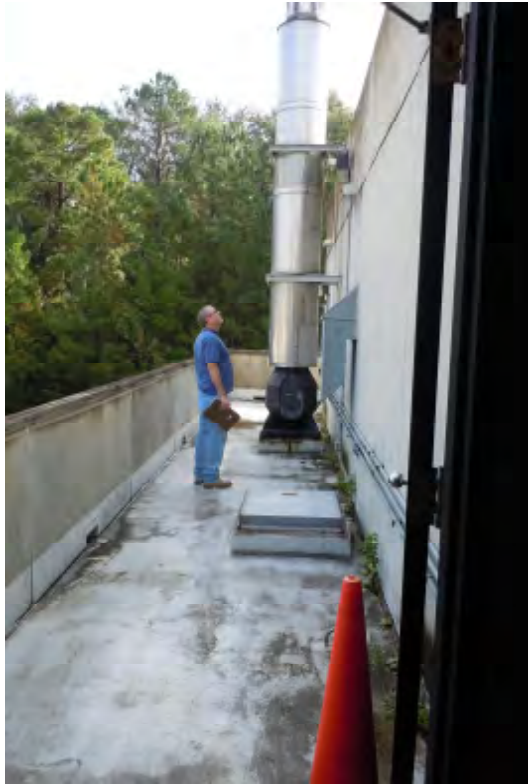
Photo #15 - Low Roof, North Side, Looking East
