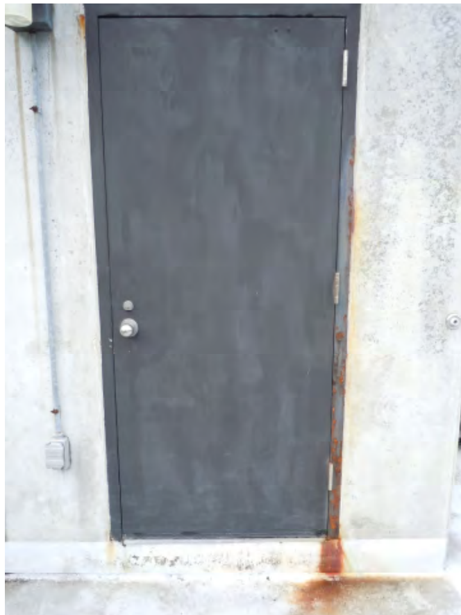
Photo #8 - High Roof, South Side
