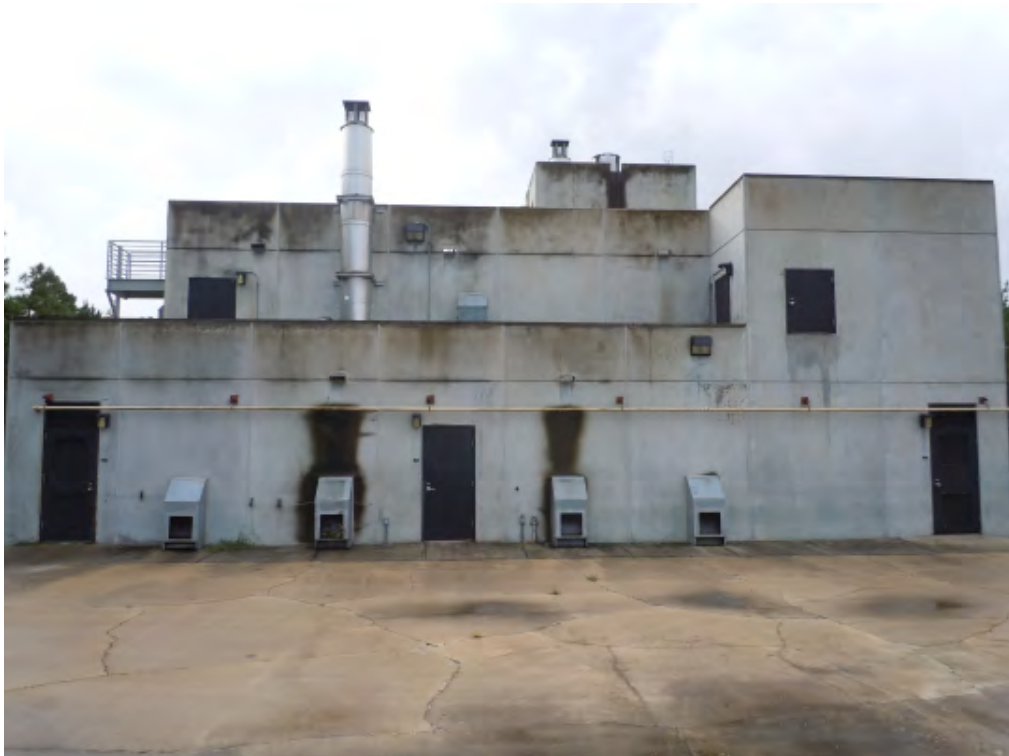
Photo #2 - North Elevation
