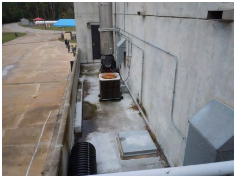
Photo #6 - Low Roof, South Side
