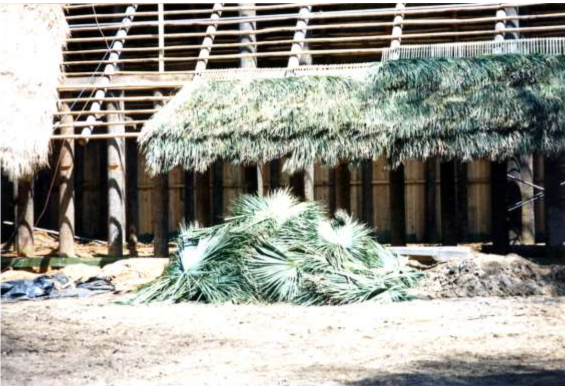
Close-up of exterior view of original thatching of 17 th century church reconstruction.
