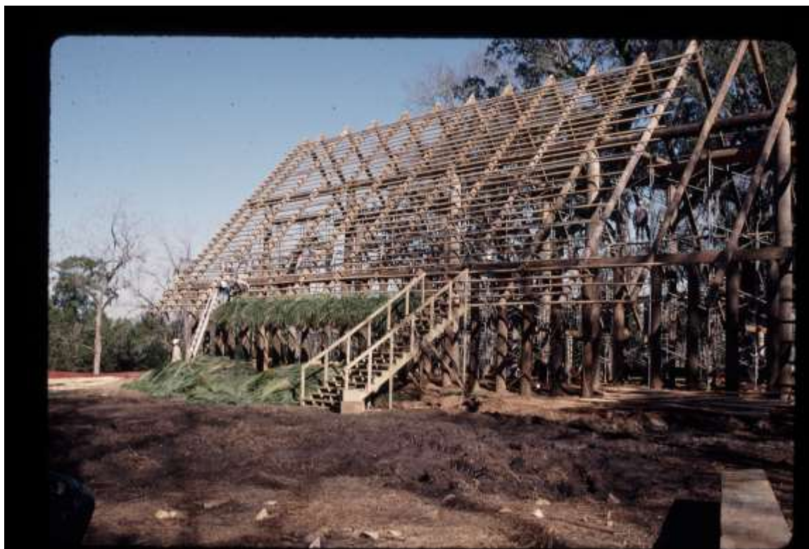
Exterior view of original thatching of 17 th century church reconstruction.
